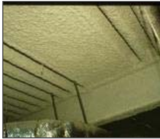
Cementitious Sprayed Fireproofing
