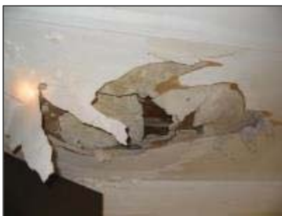
Plaster on Wood Lath
