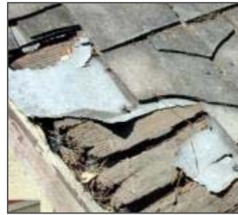
Building Paper Under Roof Tiles
