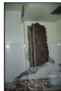
Plaster on Speed Tile
