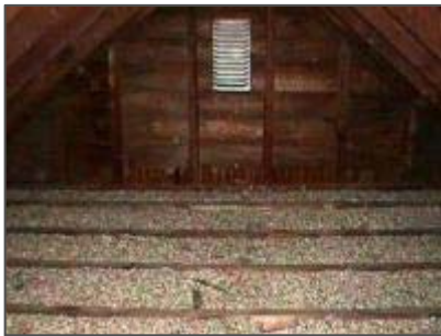
Vermiculite Attic Insulation
