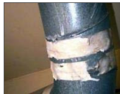
Paper on Seams of Duct
