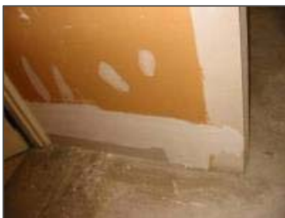
Drywall Joint Compound on Drywall
