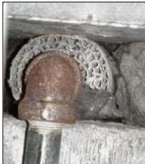
Aircell Insulation (corrugated paper)
