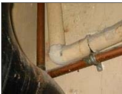
Parging Cement on Pipe Fitting
