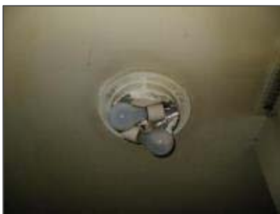
Paper Heat Shield on Incandescent Fixture
