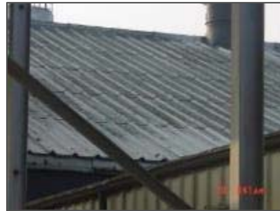
Corrugated Transite Siding/Roofing
