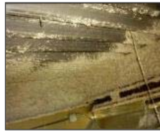
Fibrous Sprayed Fireproofing (beam only)
