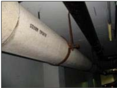
Transite Drain Pipe
