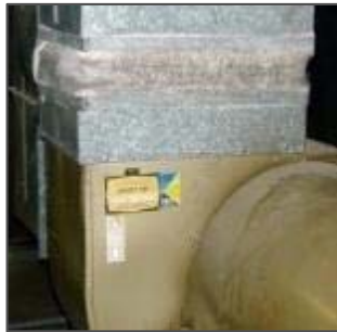
Textile Vibration Damper/Duct Connector
