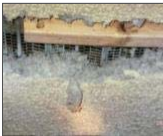
Sprayed Limpet Texture Ceiling on Lath
