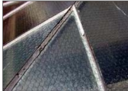
Caulking at Glazing
