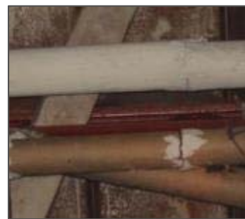
Parging Cement on Sweatwrap and Aircell
