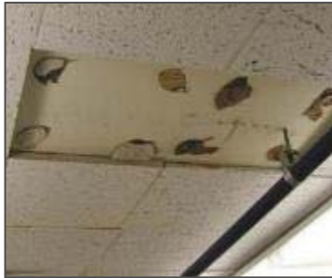
Glued on (Laminated) Ceiling Tiles
