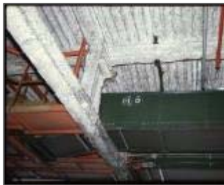
Fibrous Sprayed Fireproofing
